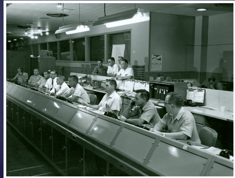
Control Central - Cape Canaveral
